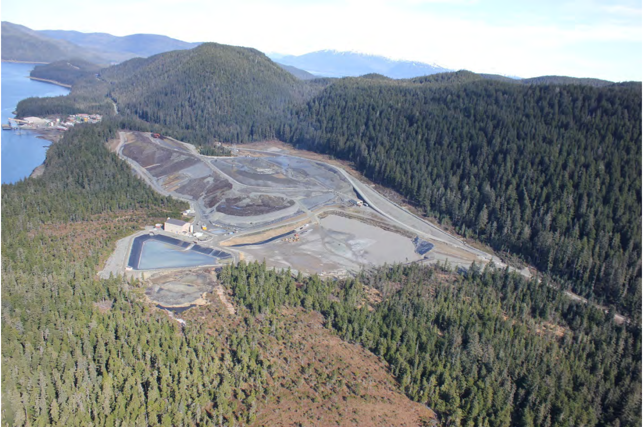
Figure 19-2. Aerial photograph of Greens Creek mining complex, Admiralty Island, Alaska.
