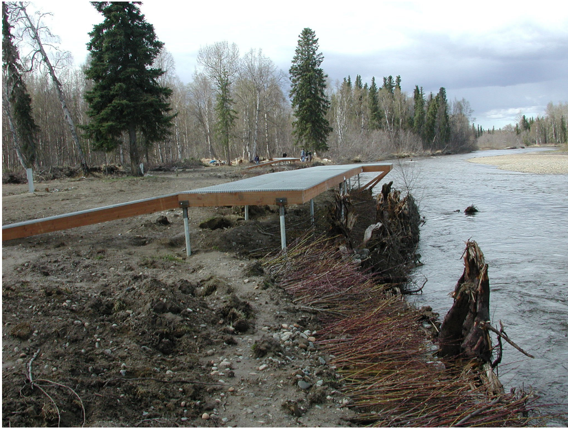
Figure A-6. Photograph showing platform construction.
