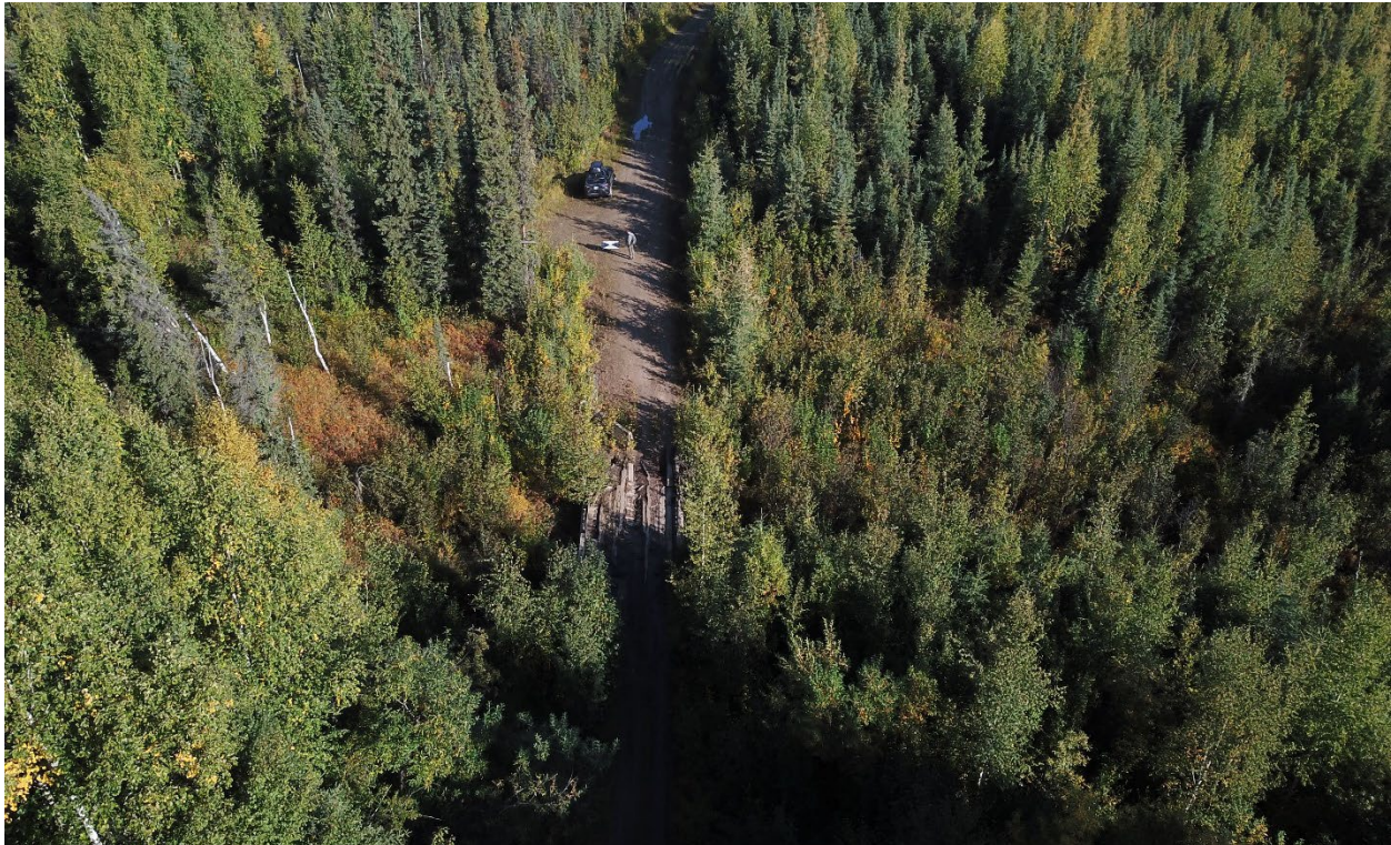
Figure 1.—September 2021 collection of additional field data. Aerial drone imagery of the existing Fortune Creek Bridge site.
