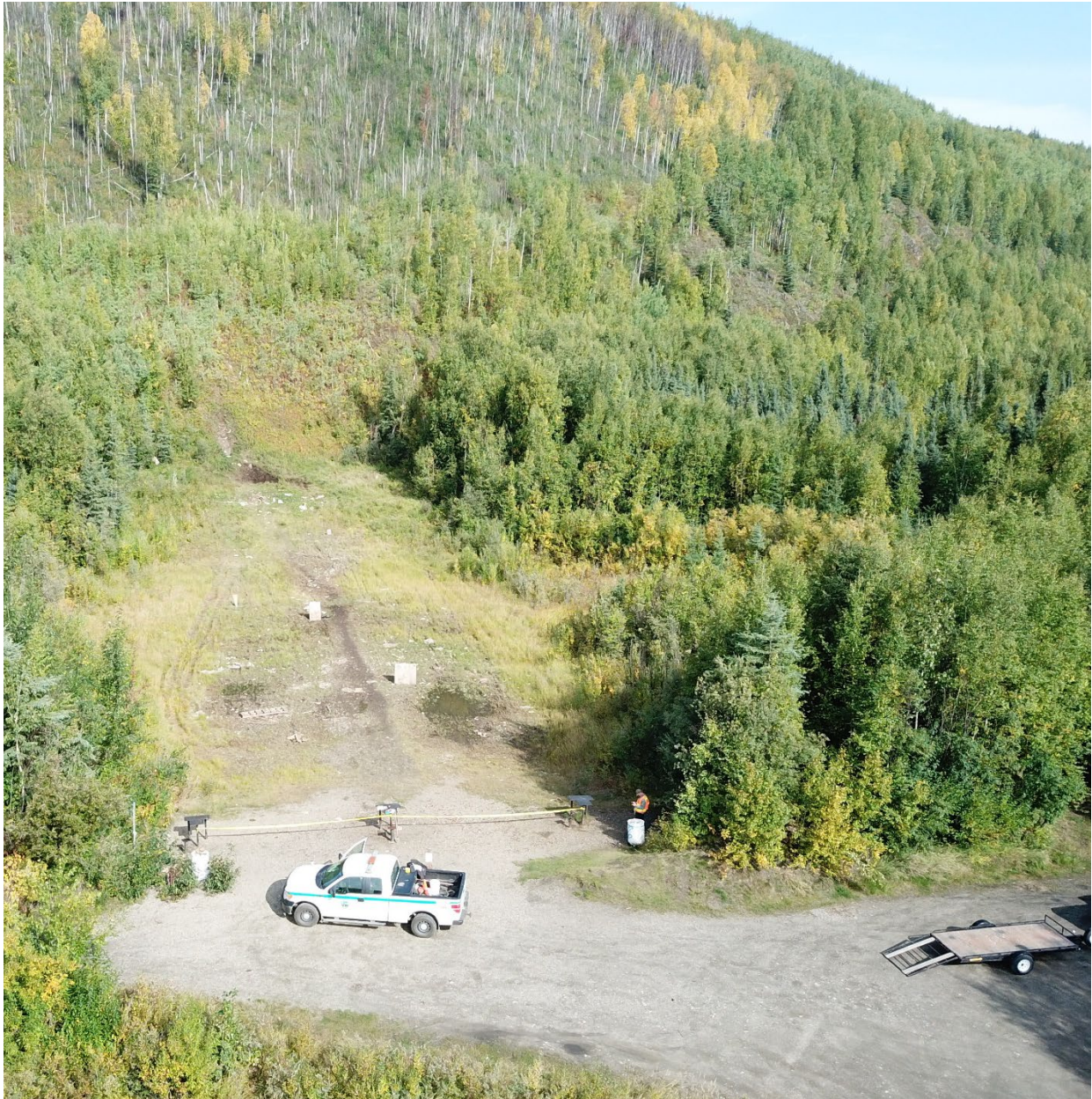
Figure 4.—Aerial view, preconstruction site visit.
