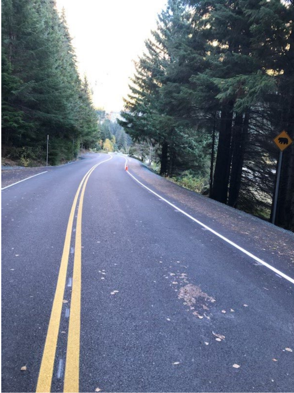
Figure 6.–Fog line striping to delineate pedestrian space.
