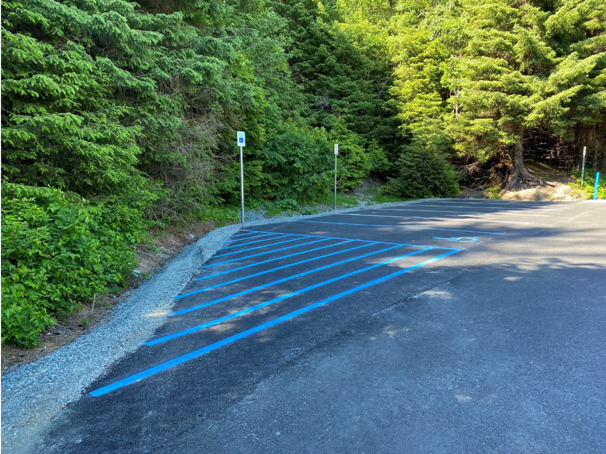
Figure 3.–Parking striping and signage.
