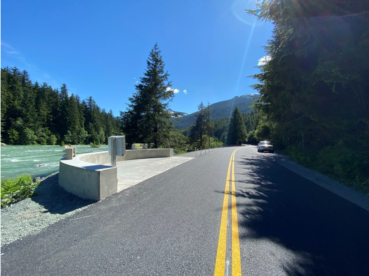
Figure 4.–Roadway striping and delineator near pedestrian area.
