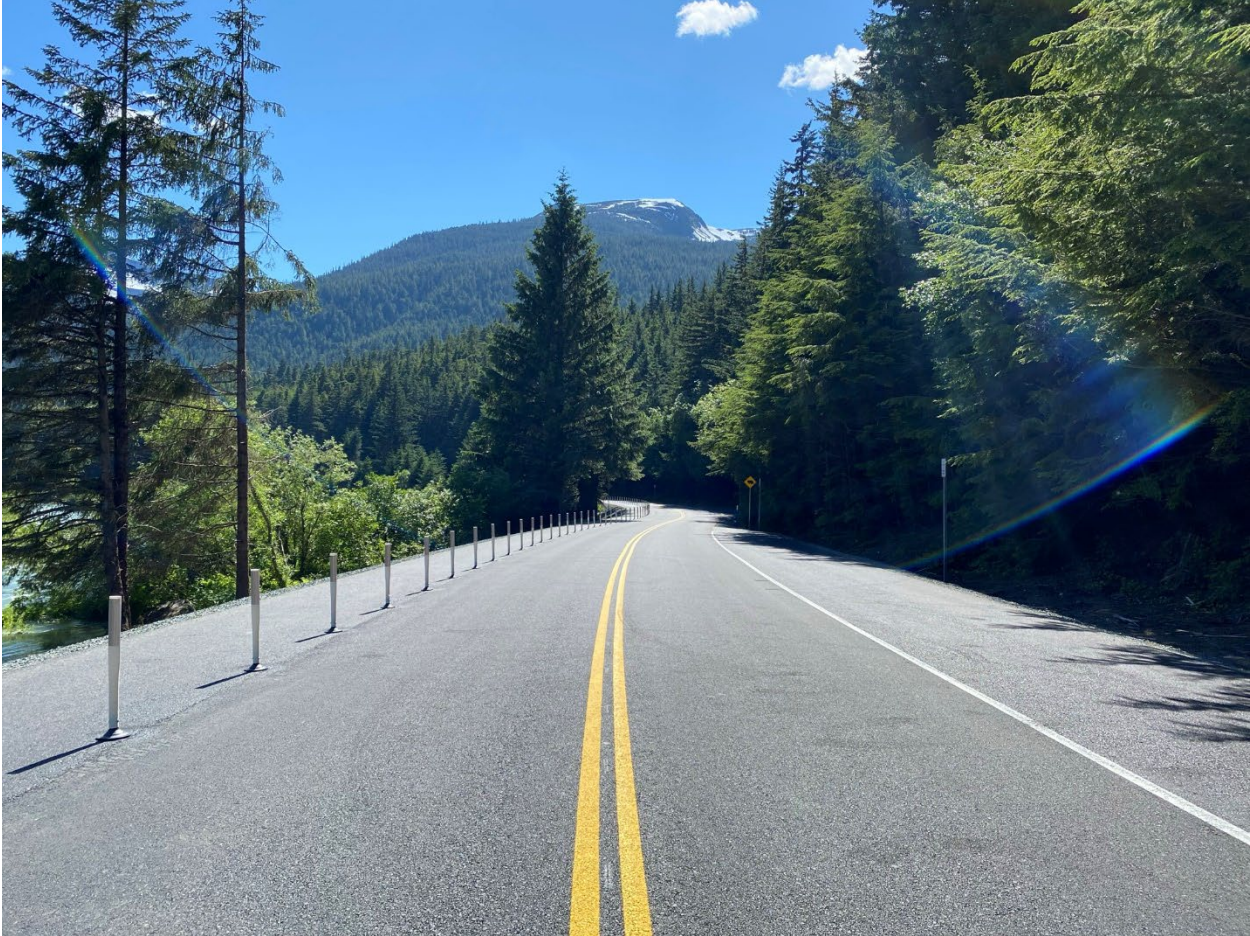
Figure 2.–Roadway striping and delineator posts.
