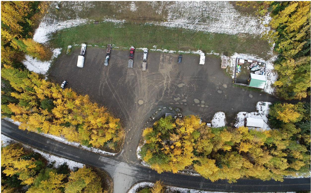
Figure 2.—Overhead drone imagery of existing Eklutna Lake TH overflow parking lot.
