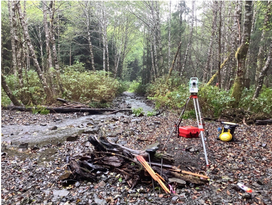
Figure 1.–Total station survey of landslide impacted areas.
