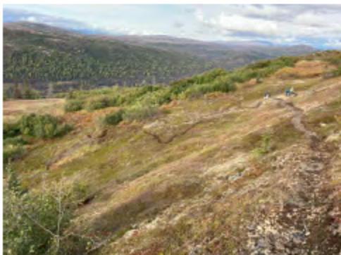
Bench cut with turns
