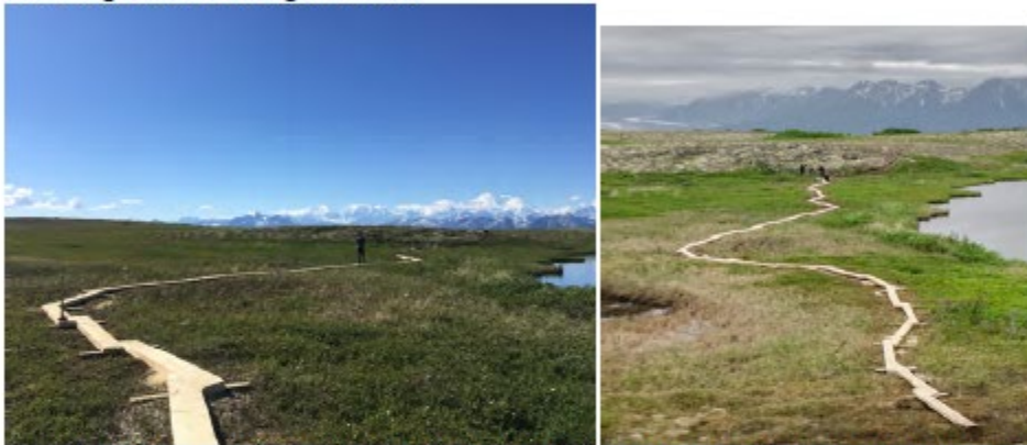
Running Plank crossing wetlands:
