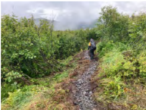
Bench cut in alder thicket w/ crush
