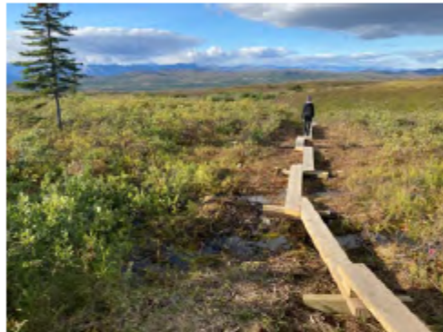
Running plank in wetland
