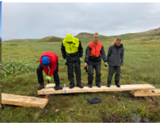
Crew setting running plank
