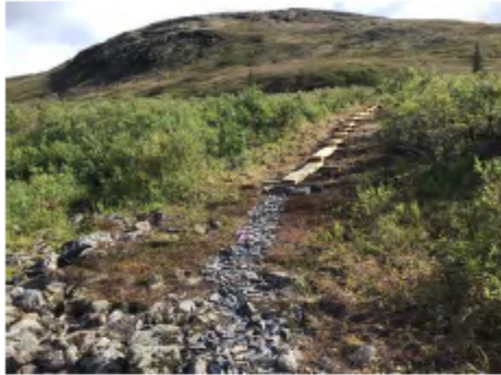
Step-and-run plank walk w/ crush
