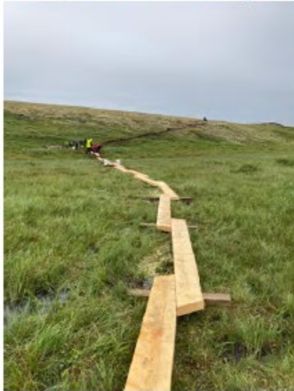
Running plank with bench cut to cairn
