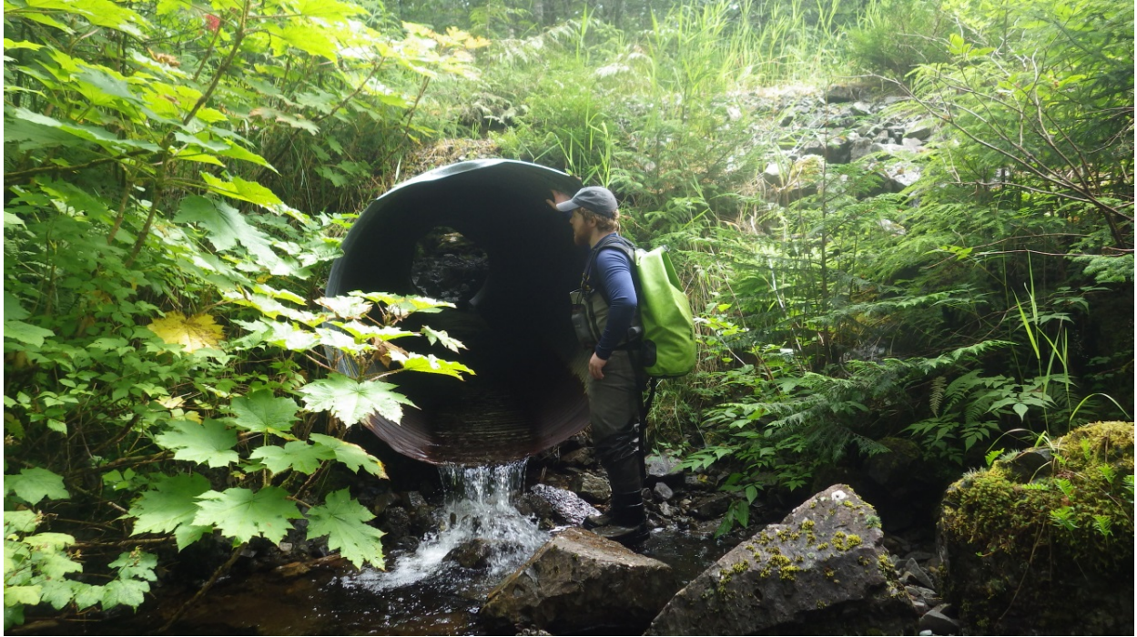
Figure 3.—Perched culvert from WPT 536.
