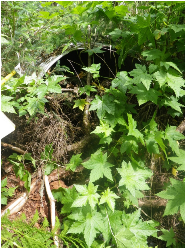
Figure 2.–Vegetation clogging a corrugated metal pipe at WPT 354.
