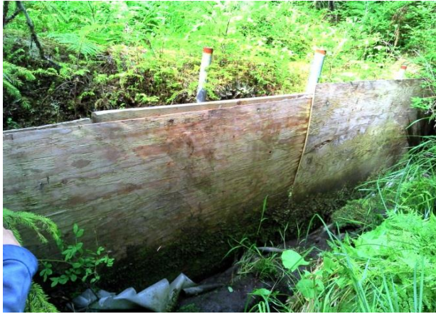
Figure 1.—Plywood structure in stream. Blocks fish passage.
