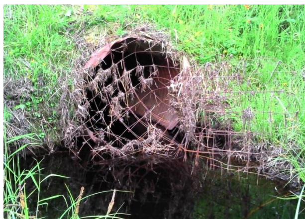
Figure 1.—Mesh wire fence on the upstream side of the culvert.
