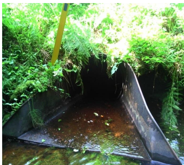
Figure 1.—Culvert outlet apron.
