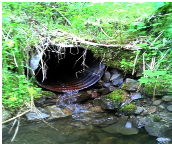
Figure 2.—Downstream side of slightly perched culvert under the boat launch road.
