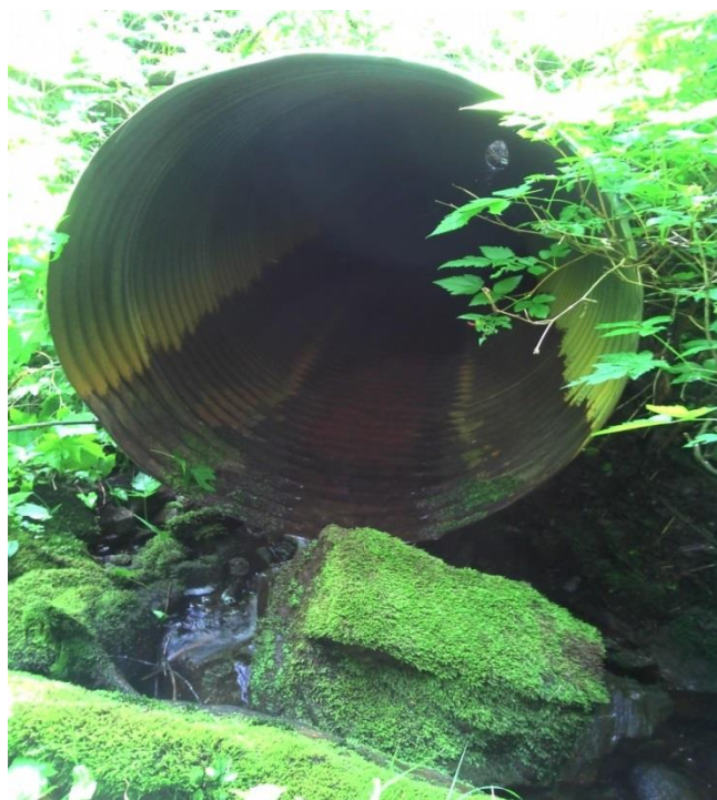
Figure 1.—Outlet of culvert perched 1.5'.
