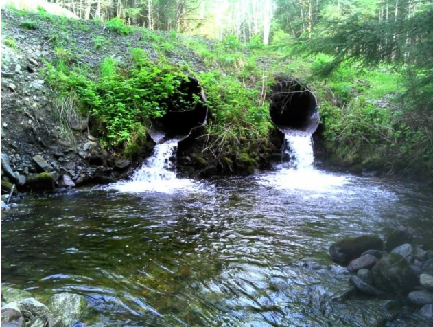
Figure 1.—Mitkof Highway 4 perched double culverts.
