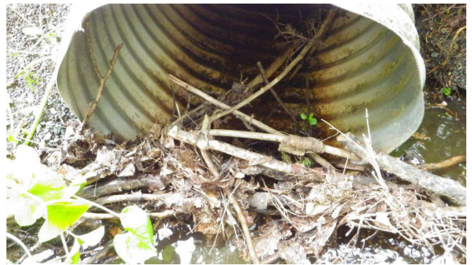
Figure 141.—Culvert filled with debris restricting flow (WPT 7).
