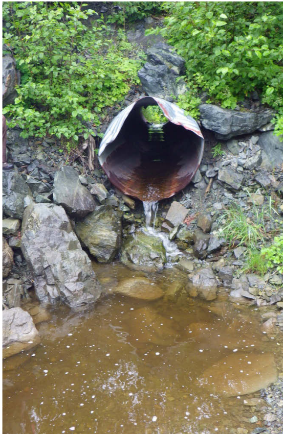
Figure 139.—Perched and damaged culvert near mouth of Cannery Creek (WPT 3).
