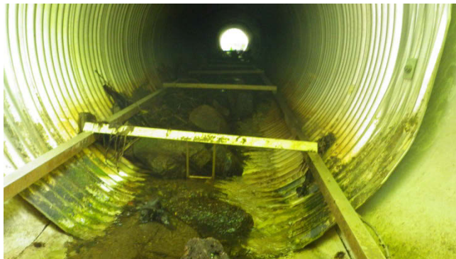
Figure 131.—Culvert beneath Mud Bay Road with fish passage modifications.
