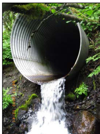
Figure 14.–Perched culvert on Falls Creek.
