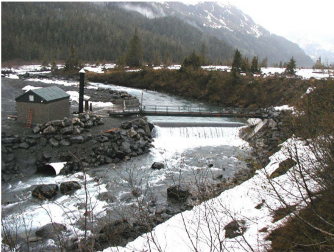
Power Creek Dam and Water Intake Photograph by Scott H. Maclean
