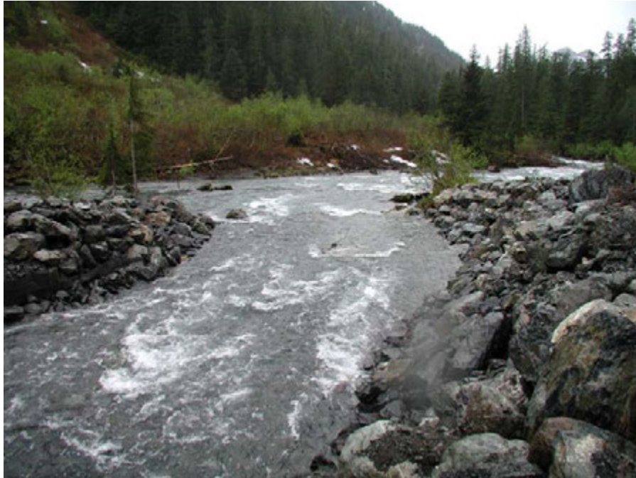
Figure 5. Power Creek Hydroelectric Project open water tailrace.
