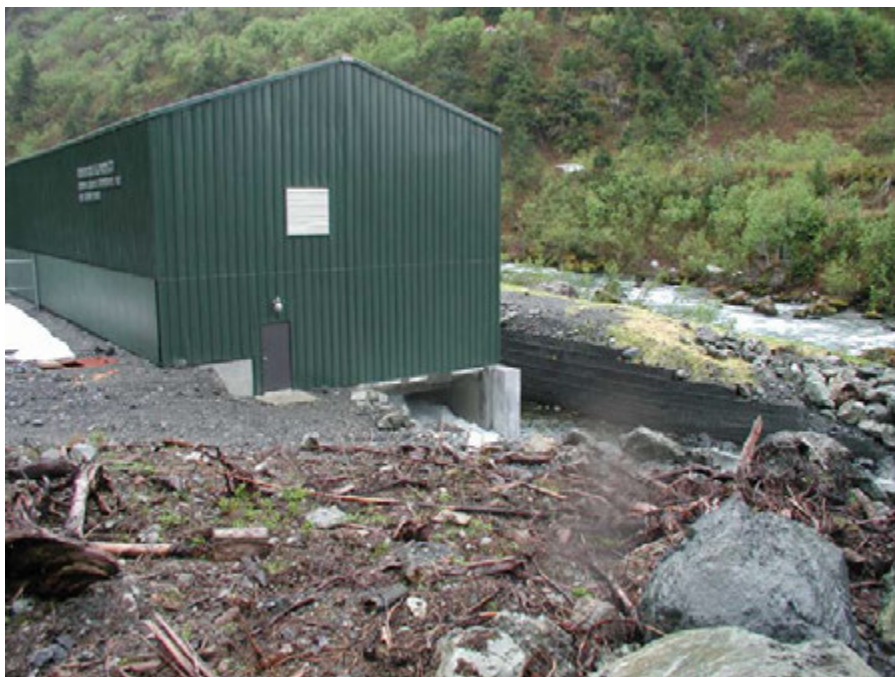
Figure 4. Power Creek Hydroelectric Project power house.
