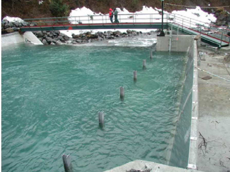
Figure 3. Power Creek Hydroelectric Project intake structure.
