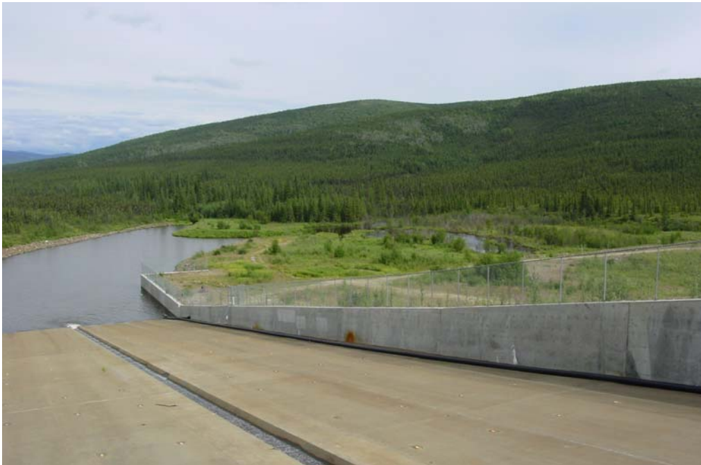
Figure 8. Spillway in Ft. Knox freshwater dam (August 2006).
