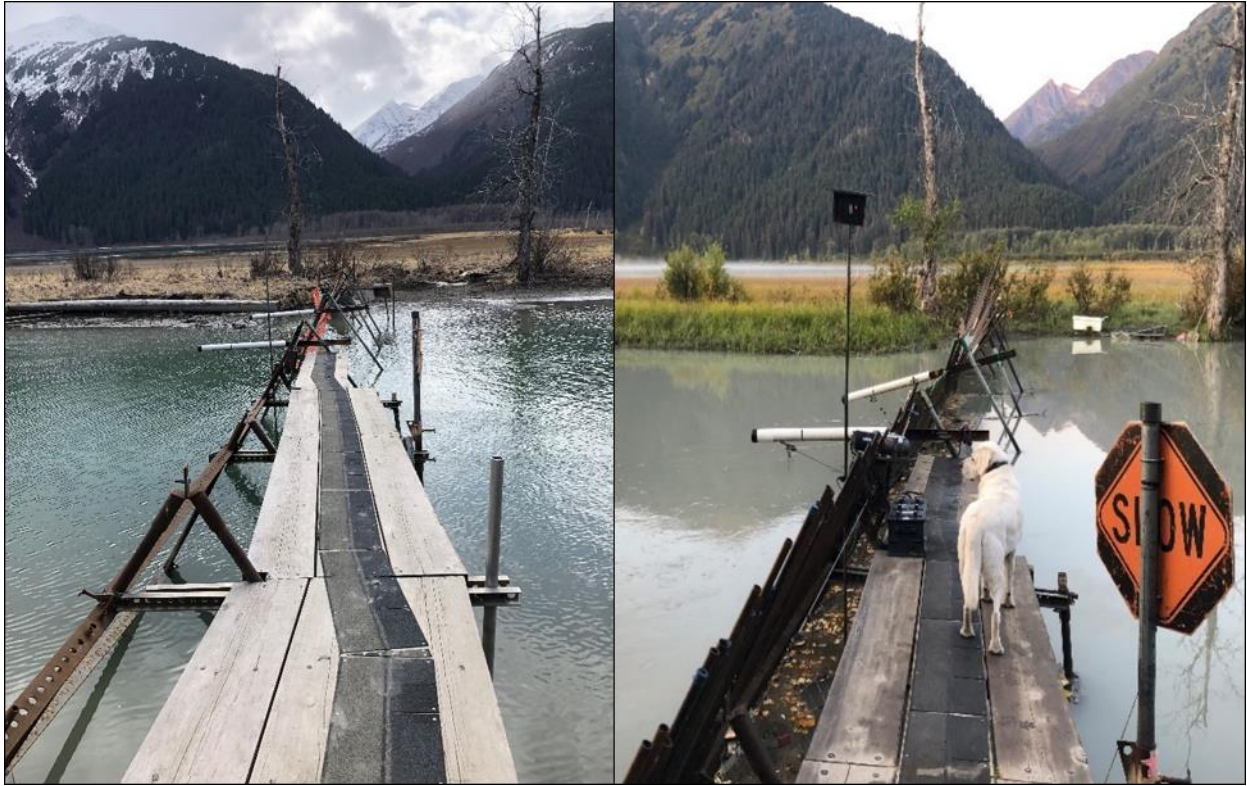
Figure 4.—Two views (from the cabin side of the creek) of the Chilkat Lake weir without pickets (left) and with pickets installed (right), 2019. (© 2019 ADF&G/photos by Nicole L. Zeiser.)
