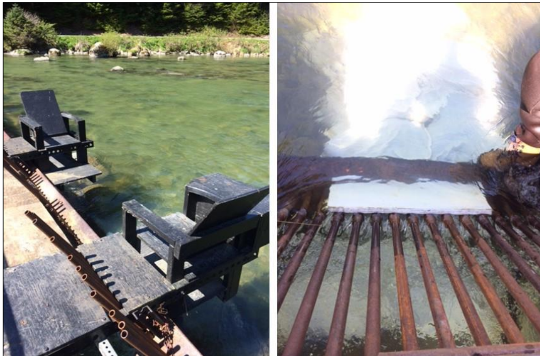
Figure 4.—Counting chairs positioned on either side of the counting station at the Chilkoot River weir (left), and opening at the counting station (right) showing where fish are counted as they swim through the weir; white plywood is stacked at the opening to force fish higher in the water column and make them easier to identify and count. (© 2019 ADF&G.)
