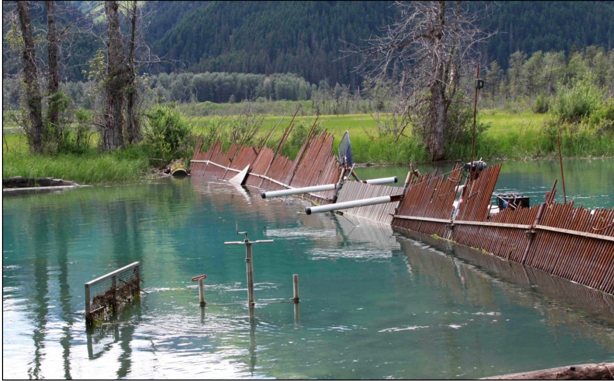
Figure 3.—Chilkat Lake weir. The boat gate is closed in the center of the weir, and the DIDSON transducer is attached to the aluminum pod visible in the lower center of the photo (©2013 ADF&G/Photo by Steven C. Heintl).
