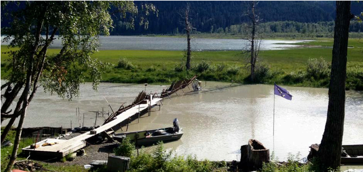
Figure 4.—Chilkat Lake weir during flow reversal, August 2014. Silty Tsirku River water is flowing from left to right into Chilkat Lake. The boat gate in the center of the weir is open to prevent damage (©2014 ADF&G/Photo by Timothy Brush).
