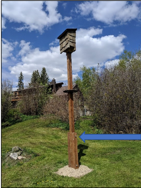
Figure 12. A jointed sectional pole to strategically hoist a bat box or rocket box. This swivel design allows one to pivot the box. It not only assists with installation but makes long-term box maintenance easier. It allows you to raise and lower the box, pivoting on the swivel point (at arrow). This picture shows a standard 4 chamber maternity box but the same approach is often used with rocket boxes. Rocket boxes are more difficult to erect, given that the chambers are built around a section of pole (see Figure 11). The section of pole that has the rocket box built around it can be of any length, with the position of the swivel varying accordingly. Photo by C. Olson.
