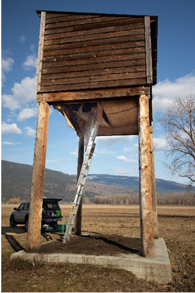
Figure 2. A bat condo, the largest type of bat house. This particular structure, built in southeastern British Columbia, uses hopper doors to enclose the roosting chambers to reduce airflow and thus increase internal temperatures. Although guano does fall onto the concrete base throughout the season, a thorough cleaning is done annually by opening the doors and sweeping out the guano deposited on the doors. Photo by J. Hobbs.
